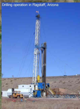
Drilling operation in Flagstaff, Arizona
